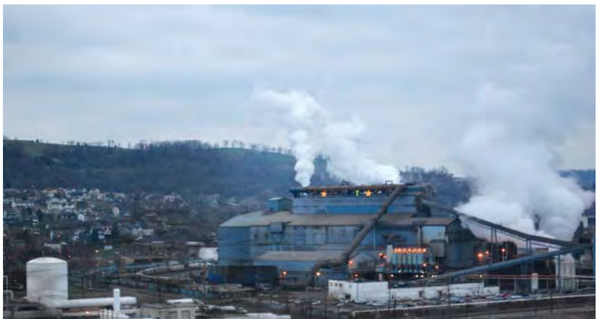
The Edgar Thompson Works steel mill, a United Steelworkers-organized mill in Pittsburgh, Pa. The mill is one of the oldest in the country.
